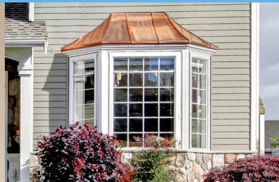
45° Bay with Copper Clad Roof
